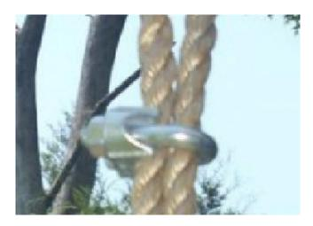
• Tighten the nuts on the U-bolt evenly using an adjustable wrench, 17mm or 11/16 wrench or socket can also be used.
